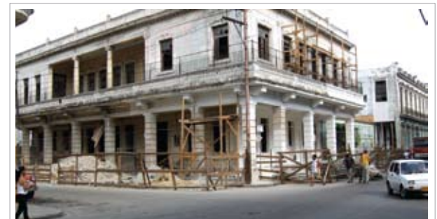
Old Club Atenas building under reconstruction as a day care center, July 2006.
